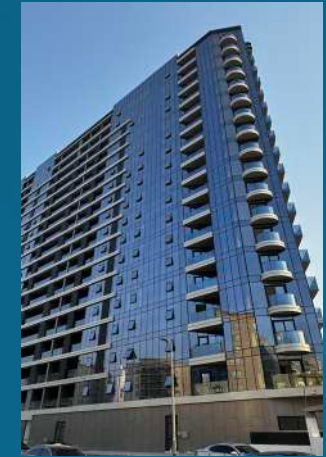
The V Tower
